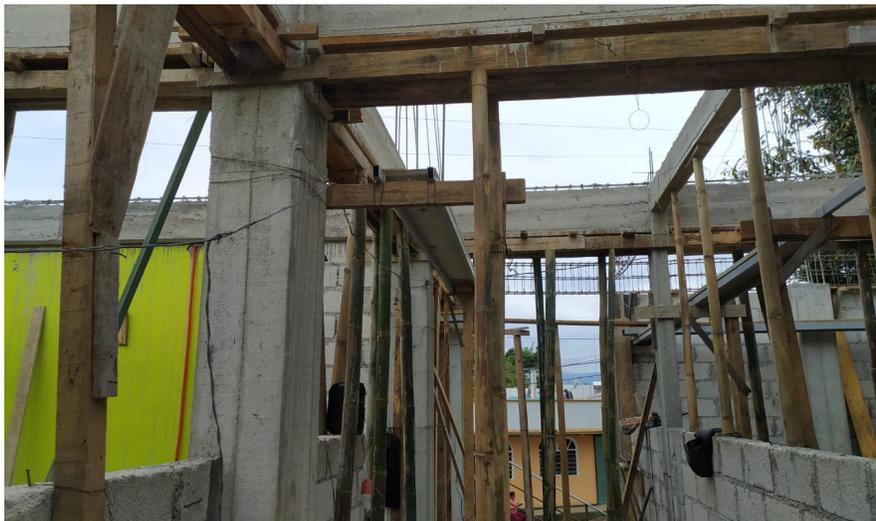
The construction crew installs girders, the main supports for the new building.
